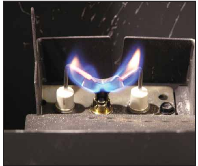
Figure 3.1 IPI Pilot Flame Patterns
