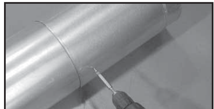
Figure 8.8 Screws into Slip Section
